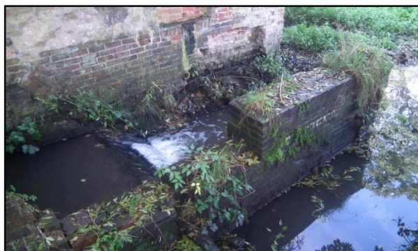
Mancetter Mill - Mill-race and Wheel pit
