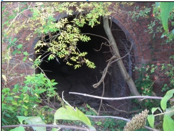
Tunnel to Jee's Crushing Plant from Jee's Quarry. [Access courtesy of John Styles (Security Manager)]
