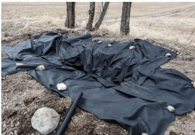
The hole was then lined with geotextile...
