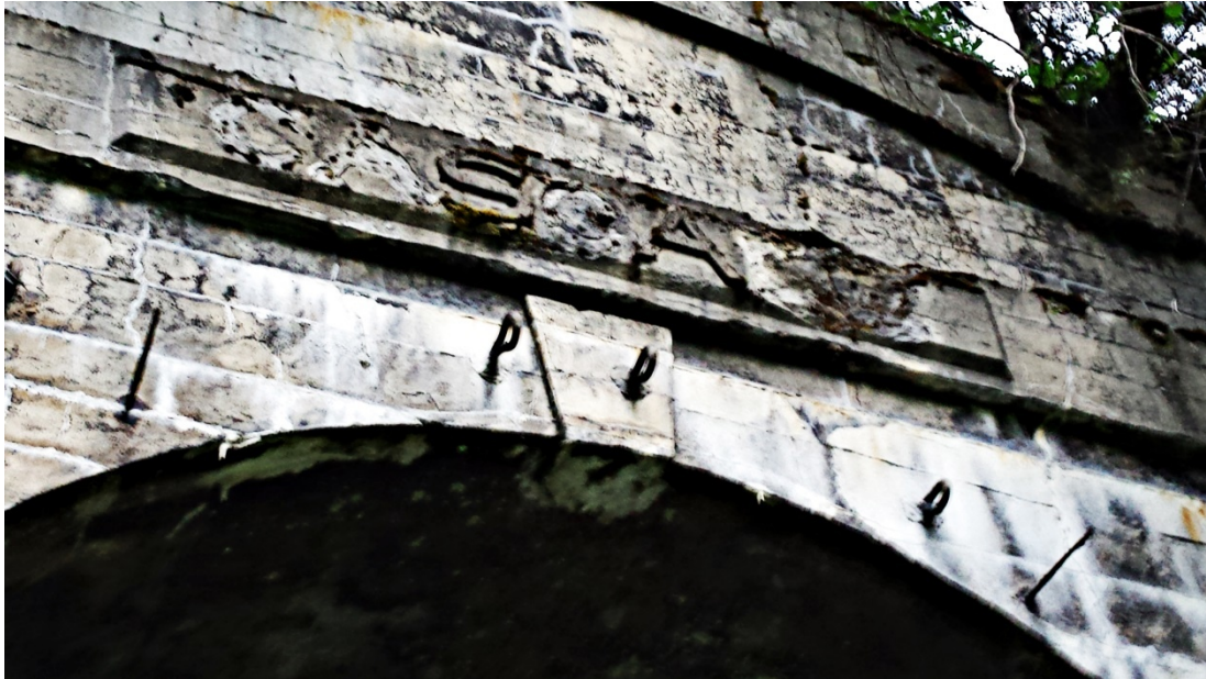
The name of the Cascade Tunnel is still visible over the portal. Hooks held electrical wires to power fans.
