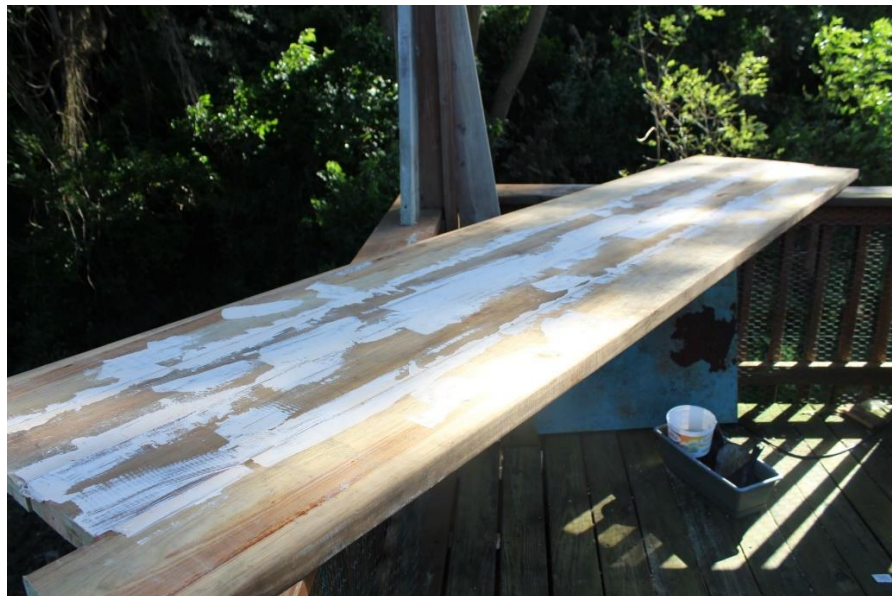
First filler in place
